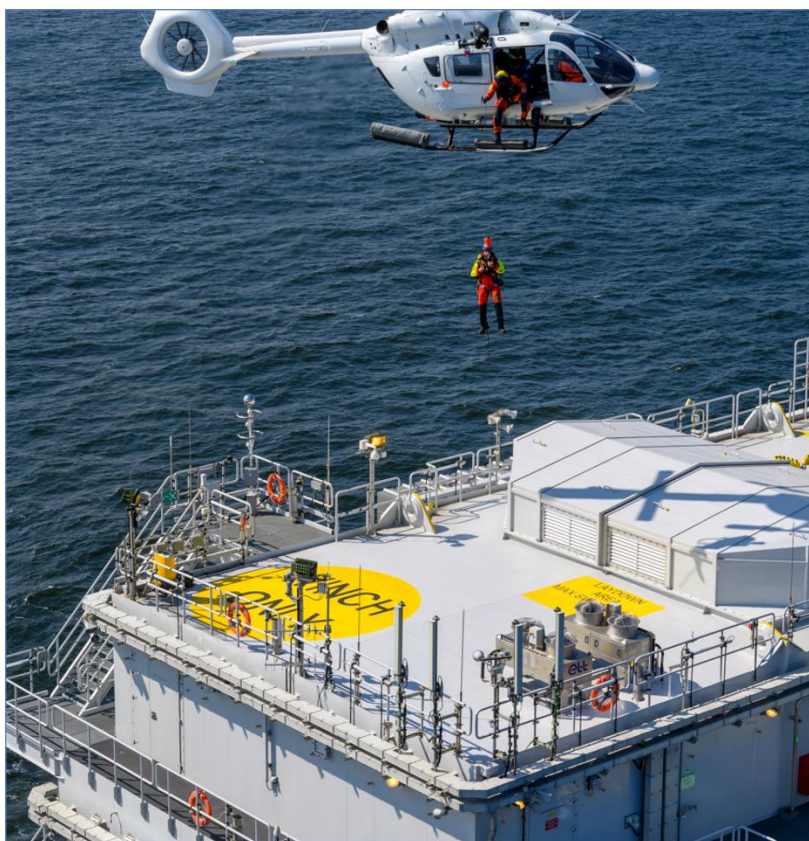
Figure 11-1: Example of Helicopter Hoist Area (HHA) on Offshore Sub Station (OSS) (Courtesy: NHV, Tom Buysse)
